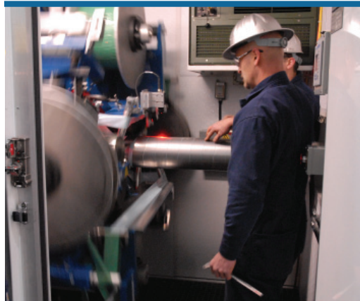
Application of UHSS reinforcement
