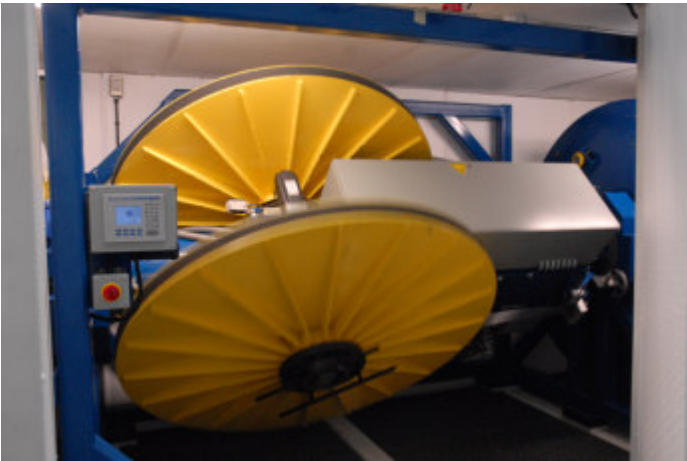
Figure 2&3 - Steel strip forming & Pay-off reels
